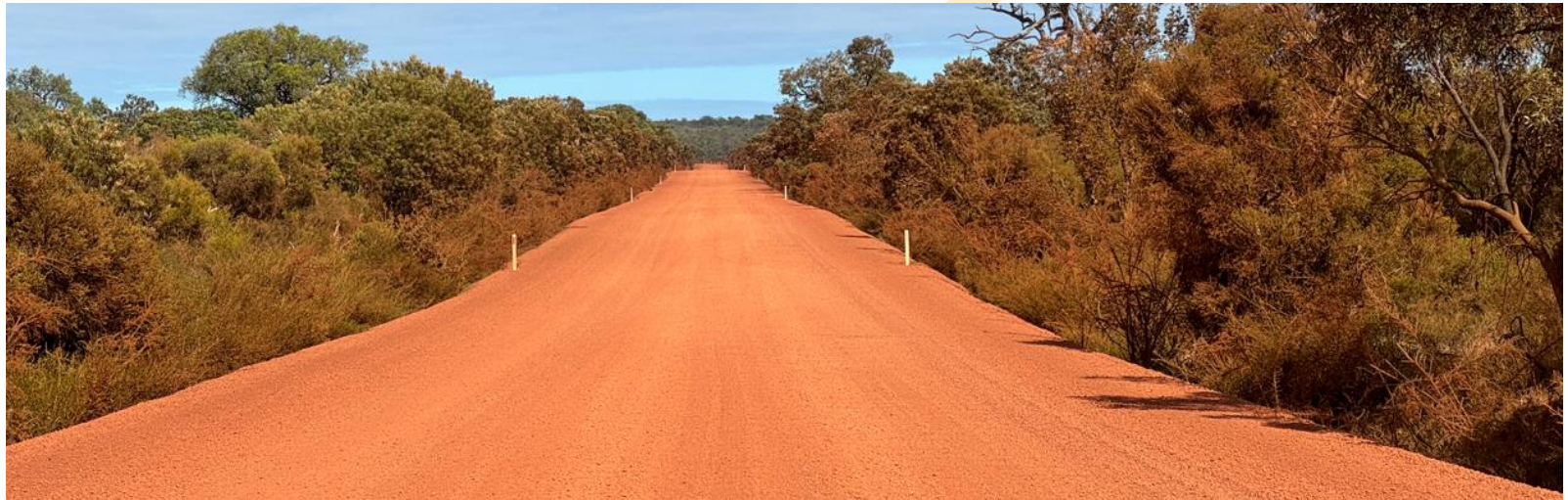
Photograph 2 – Typical layout of unsealed section of Wannamal Rd West (12 March 2024)
