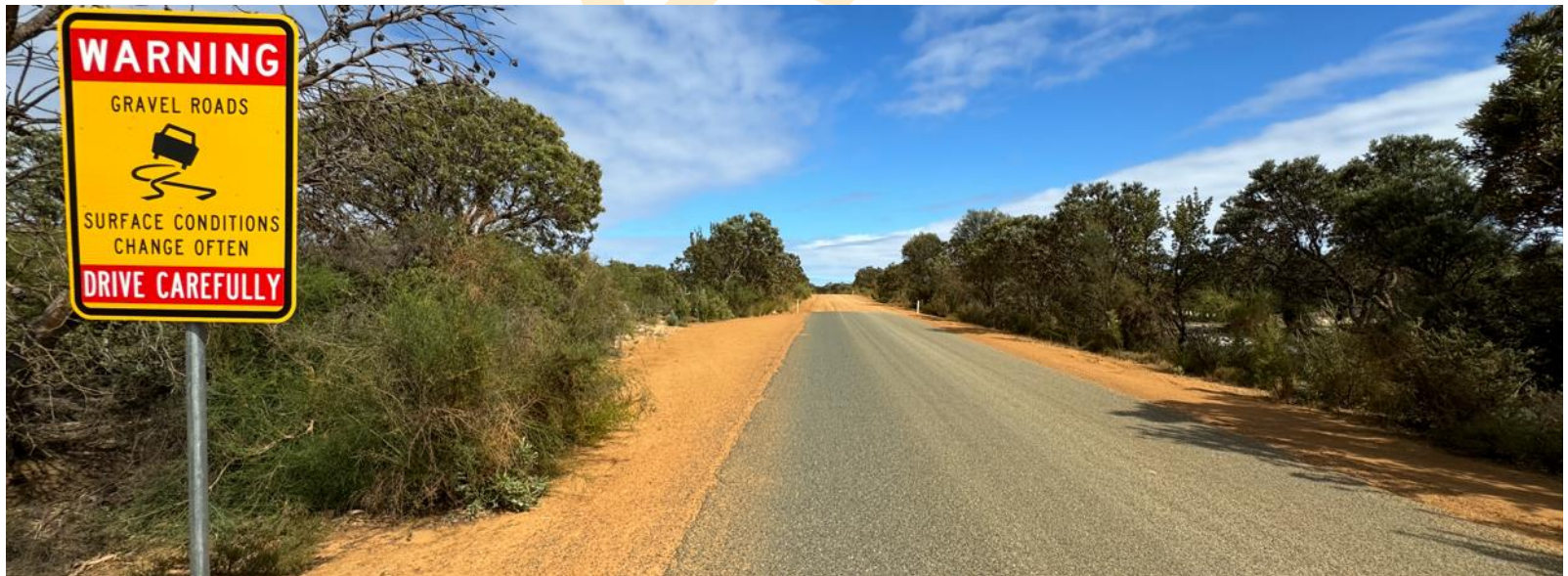
Photograph 3 – Typical layout of sealed section of Wannamal Rd West (12 March 2024)
