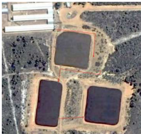
Figure 1. Mindarra 3 Wastewater Treatment System
