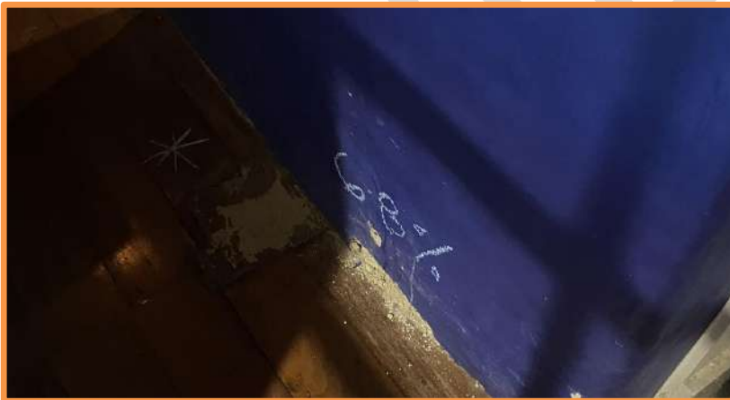
Figure 2n_2: - Timber Planks to another area;
