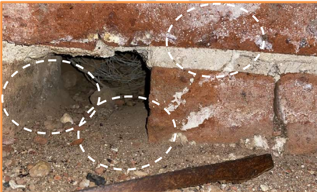
Figure 2j: - Existing Floor under server area
