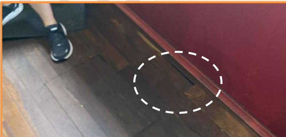
Figure 2I_1: - Existing Floorboard to main server area;
